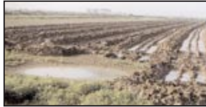
Figure 4. After pond bottom sediments become firm enough to flow, use a dozer to row up the material.
